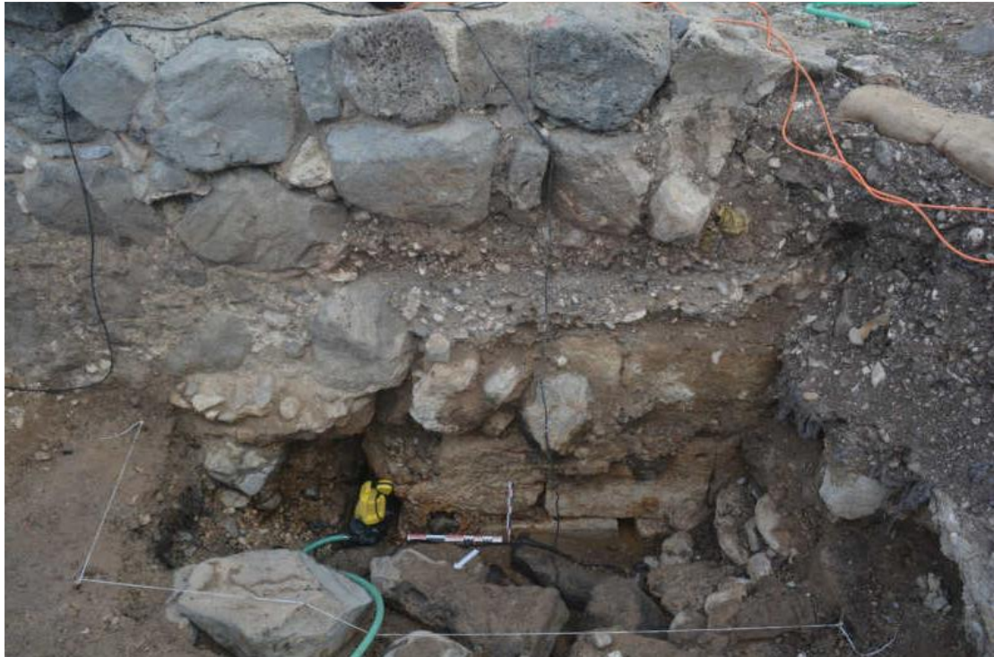
Figure 4. Junction between the W1002 (basalt wall) and the w1001 (limestone wall) (Photo by E. Nantet 2021)
