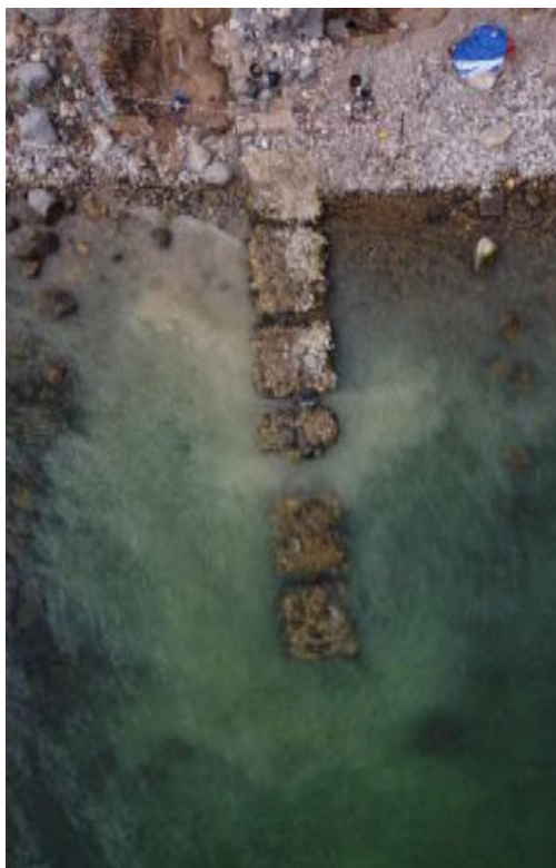
Figure 5. W1003 (Concrete pier) (Photo by J. Kim)
