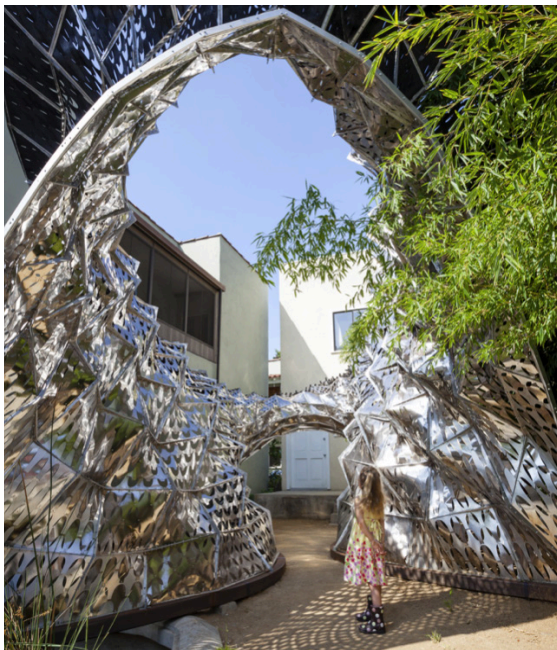
Figure 19: Bloom, made out of a 'smart' thermal bimetal is a sun-tracking instrument indexing time (Sung).
