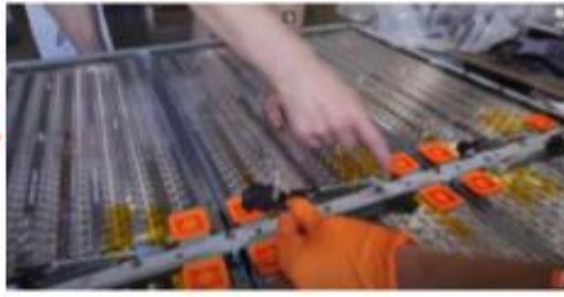
Taking out BMS wiring
