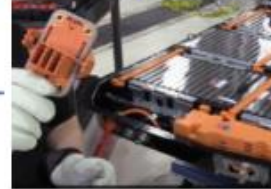
disassemble high voltage DC connector
