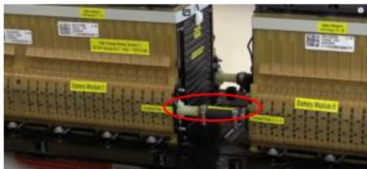
Connect the cooling passage
