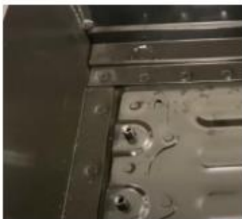
self piercing rivet attached to the battery tray
