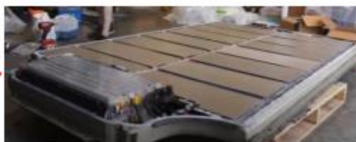
After removal of top cover
