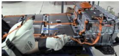
Disconnect High voltage battery cell monitoring circuit
