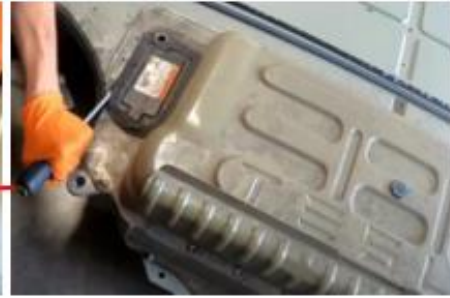
Taking the fuse box out, mounted with 9 bolts
