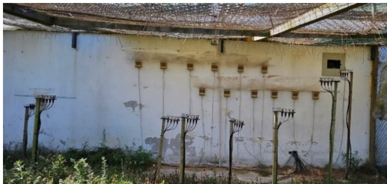
Figure 1. Placement of the 12 feeders in the mesocosm.
