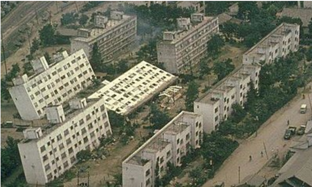
Figure 2.4: Liquefaction-induced damages illustration –tilt of building after 1964 Niigata earthquake (Kramer, 1996)
