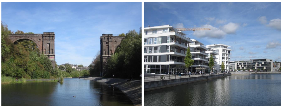
Figure 4: Phoenix, Dortmund: Viaduct Hympendahlbrücke (Eliasbahn) (left). Phoenix See urban development, partial view (right). Source: E. Asprogerakas.
