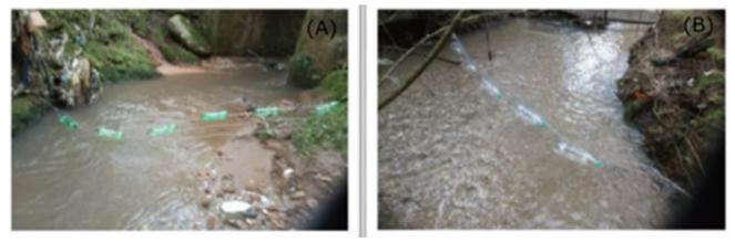
Figure 3 Ecobarriers in water bodies: A. Ecobarrier 1; B. Ecobarrier 2.
