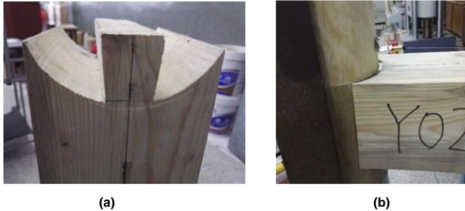
Fig. 8. Damages of dovetail tenon joints: (a) Deformation of dovetail tenon; (b) Residual length that tenon pulled out of mortise
