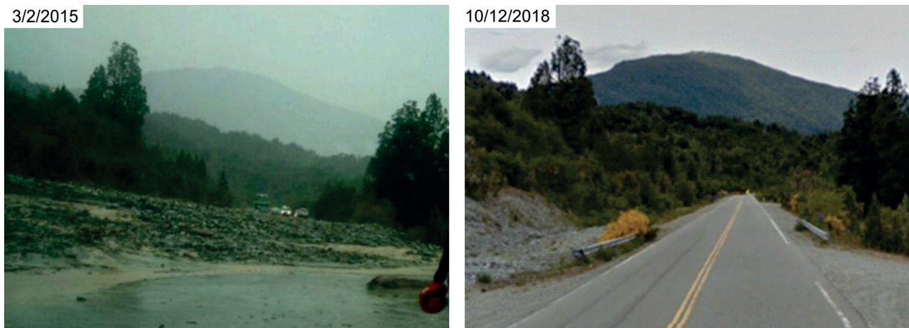
Figure 2. Debris flow event in La Cantera watershed that generated a roadblock on National Route 40 (3/2/2015). Source of the left image Digital Newspaper Bariloche 2000. Right image taken by the authors.
