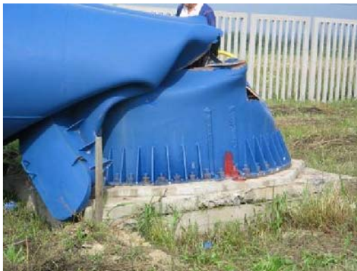
a) breaking the water tower at the root pole
