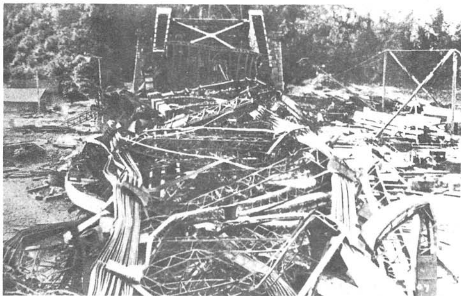
Figure 7(a) Wreckage, looking south [top]; 7(b) looking north
