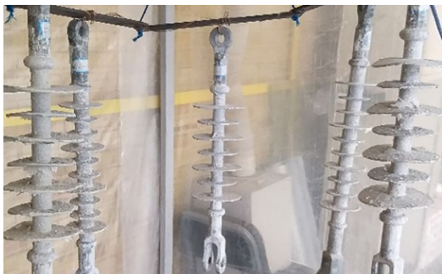
FIGURE 2 The polluted insulators and pollution process.
