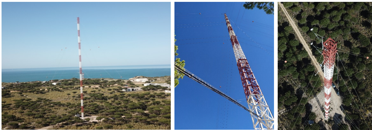
Figure 8. El Arenosillo tower where GHG concentrations and meteorological parameters are measured at 10 m, 50 m and 100 m.
