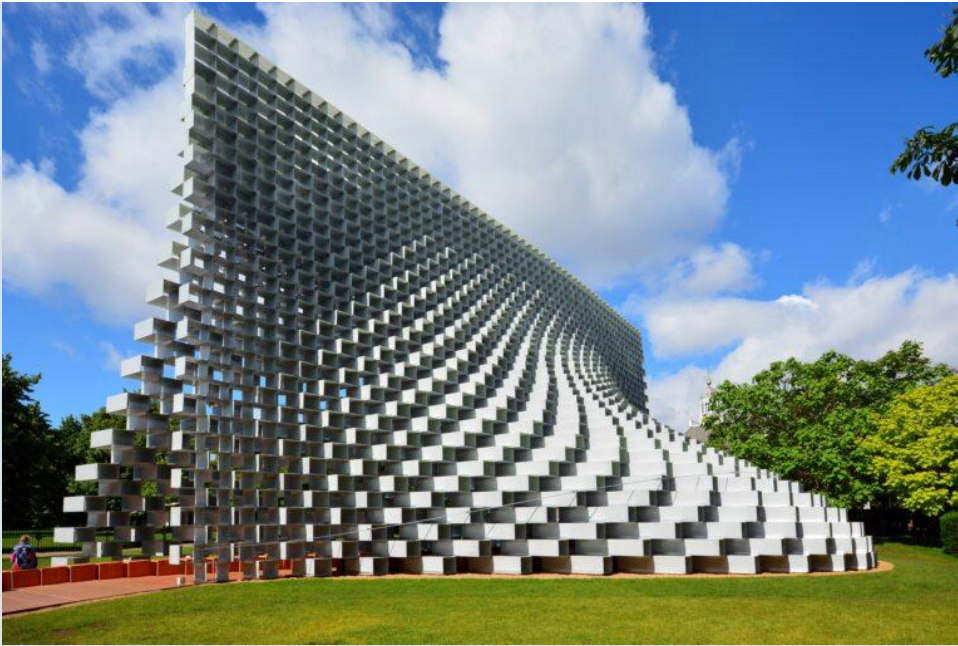
Figure 6. Serpentine pavilion 2016 by BIG. Source: George Rex (permission granted).
