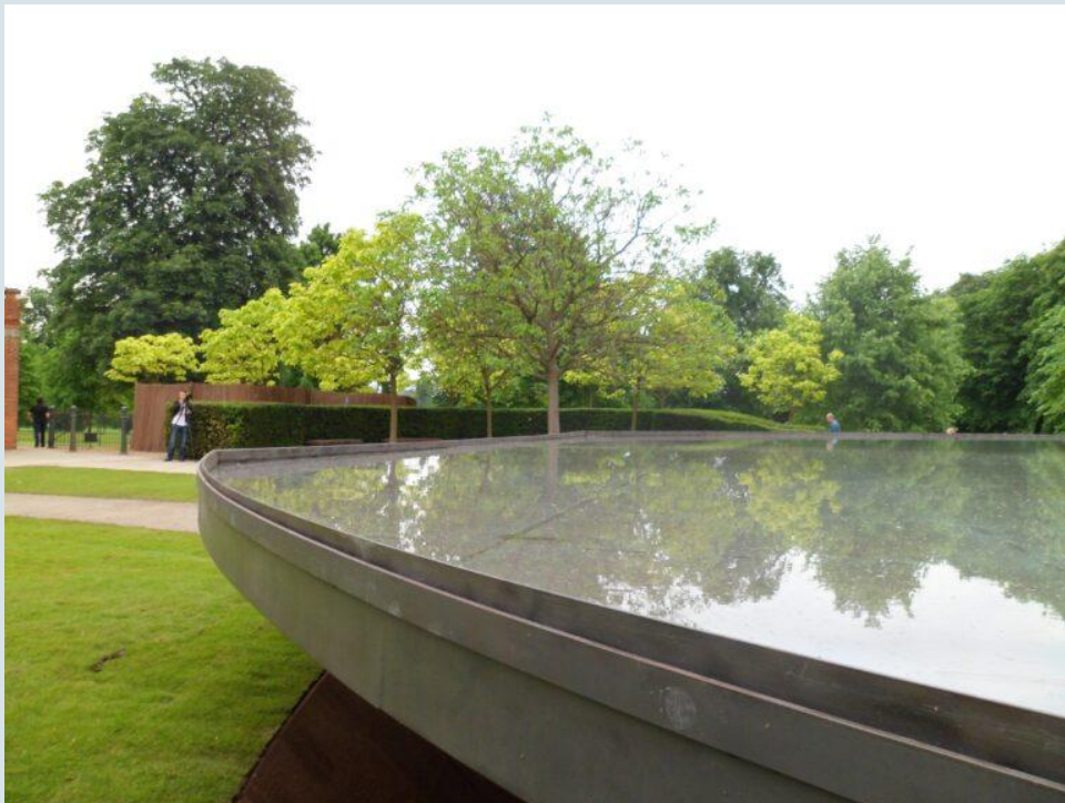
Figure 9. Serpentine, roof containing a shallow pool of water. Source: Author.
