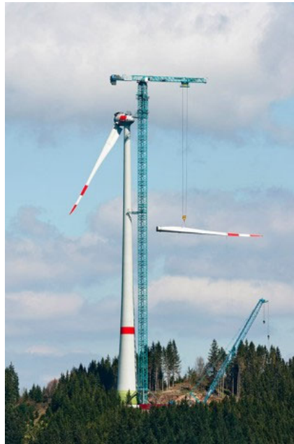
Figure 1-2 Litronic tower crane erects a wind turbine (Wind Power Engineering, 2016)
