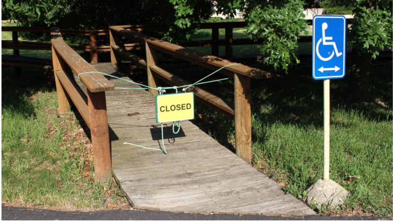
Figure 10 The image is one of the entrance ways to the accessibility ramp and its exemplar “Closed” sign and rope barricade at one of three entrance points to the accessibility ramp.
