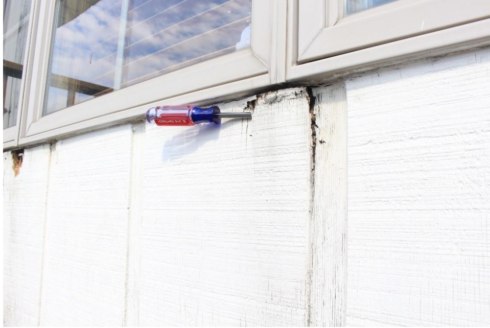
Figure 18 This image is a closer look at the siding and the siding is deteriorating beneath the vicinity of the triple mullion dining room window. The screwdriver is inserted in the decayed area to indicate that the area is deteriorating.
