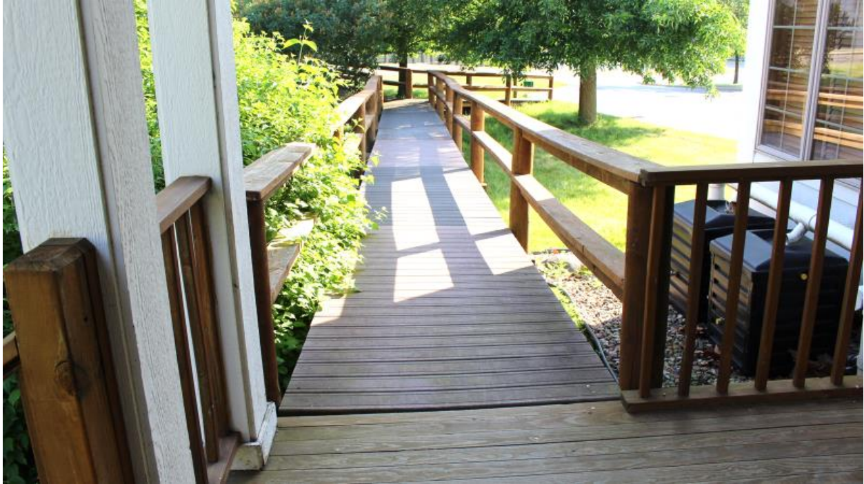
Figure 11 This image of the accessibility ramp from the front porch view. The images shows that the area should have a closed sign as in figure 10.
