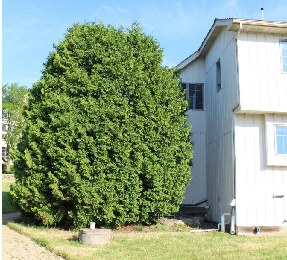
Figure 19 This image is a large cedar tree near the house, which is located on the Southwest side of the house where decay may be accelerated because of the tree due to the fact that there's not enough sunlight which means more moisture is acceptable in this area.
