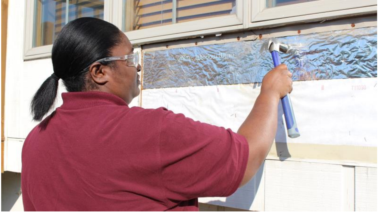
Figure 21 This image is illustrating the student using a hammer gently striking silver area underneath the side to determine if moisture is present.
