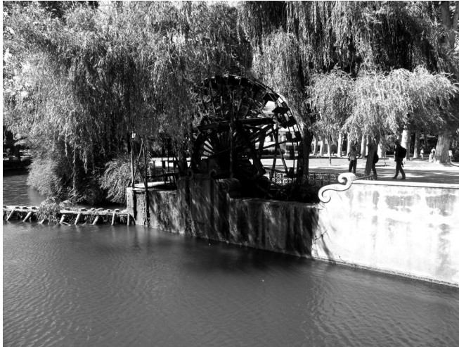
FIGURE 6 The vertical water wheel of Mouchão in Tomar
