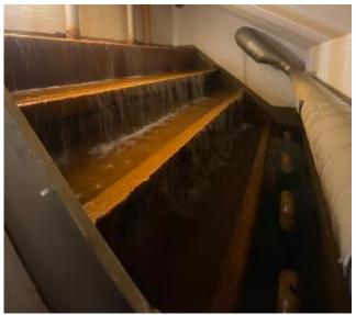
*Figure 7.5 Picture taken from one of the two cascade aerators in Hinnerup during the visit in the waterwork on the third of May.*
