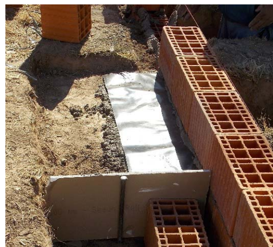
FIG. 6 POLYETHYLENE FILM TO ENSURE THE WALL-BARRIER JUNCTION
