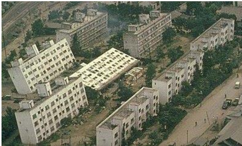
Figure 2.3. Bearing capacity failure due to Niigata earthquake, 1964.
