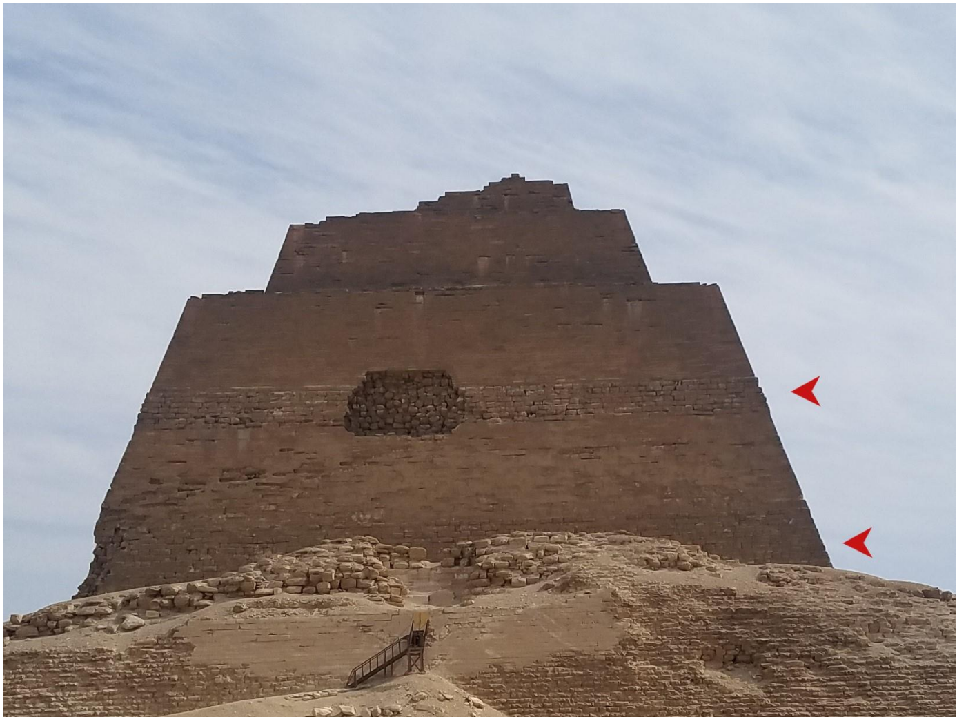
Figure 27: Meidum Pyramid showing two strips of rough masonry (photo by author).
