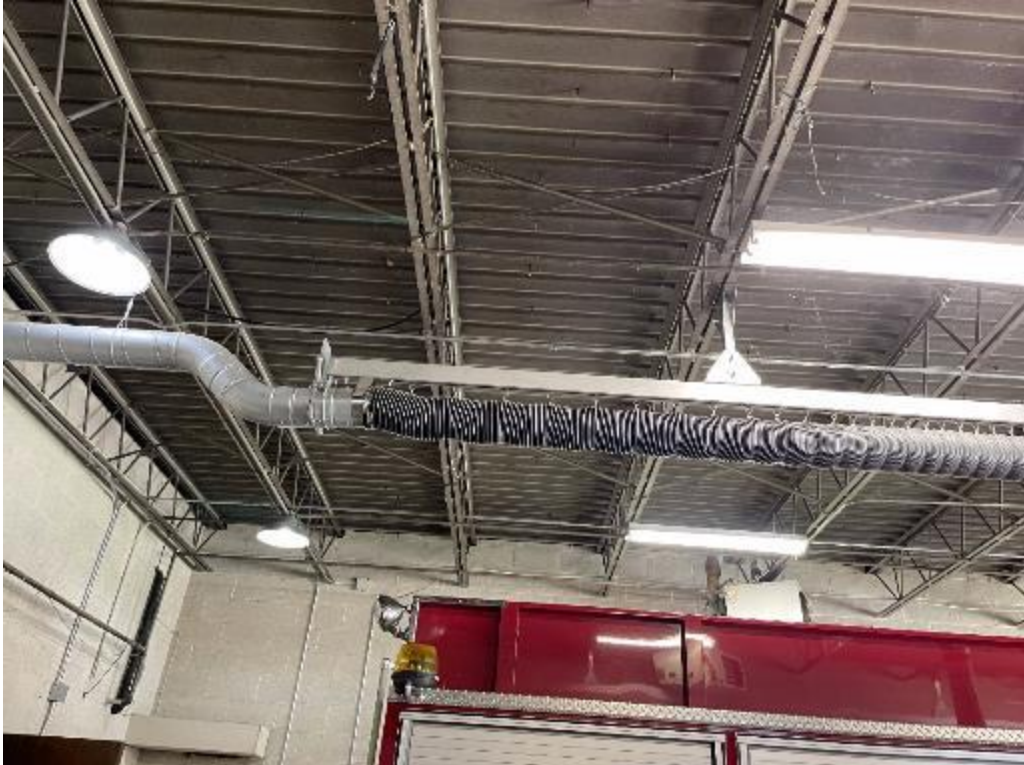
Figure J.29 Image of Structure #21
