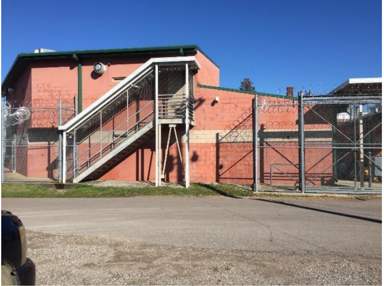
Figure J.8 Vertical Irregularity in Structure # 3.3
