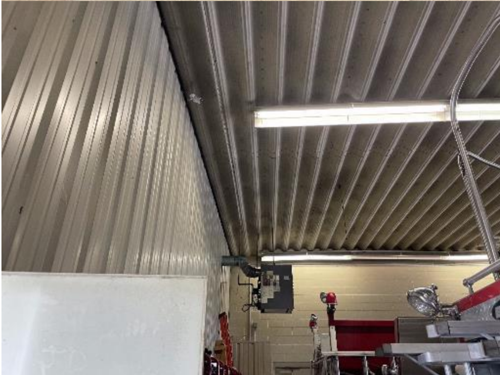
Figure J.21 Image of Structure #19.1
