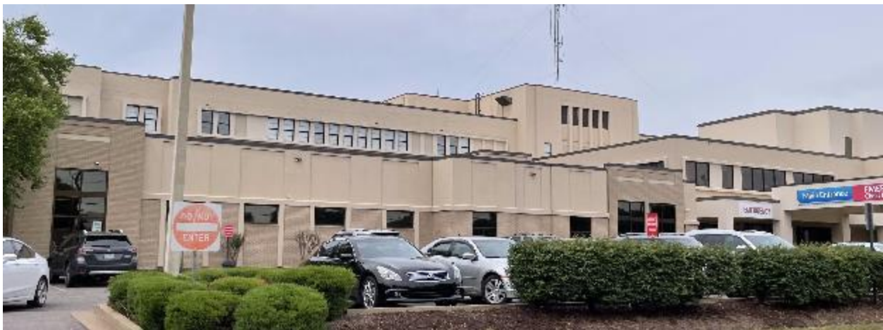
Figure 3.22 Out-of-Plane Setback Vertical Irregularity from Site Visit
