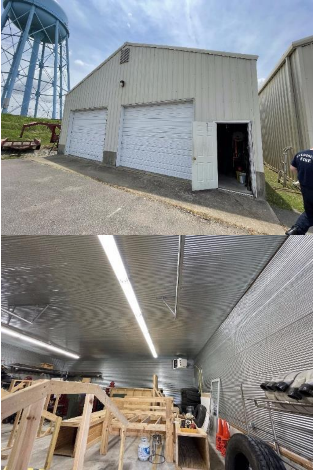
Figure J.25 Image of Structure #19.3
