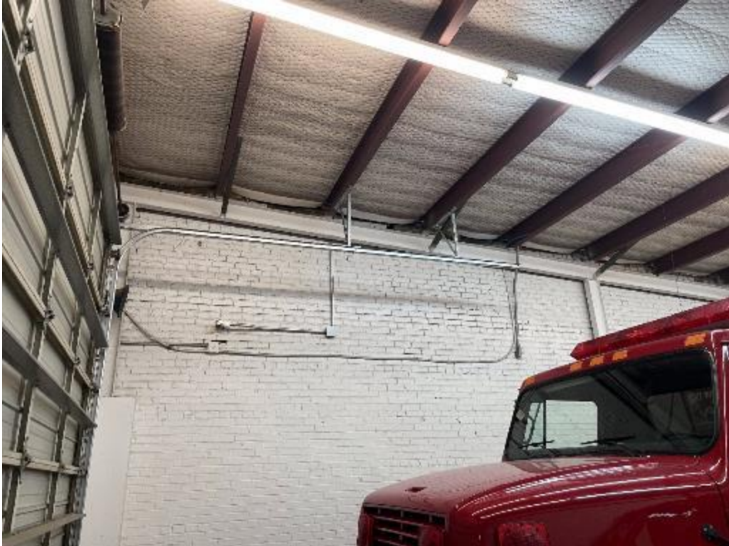
Figure J.27 Image of Structure #20
