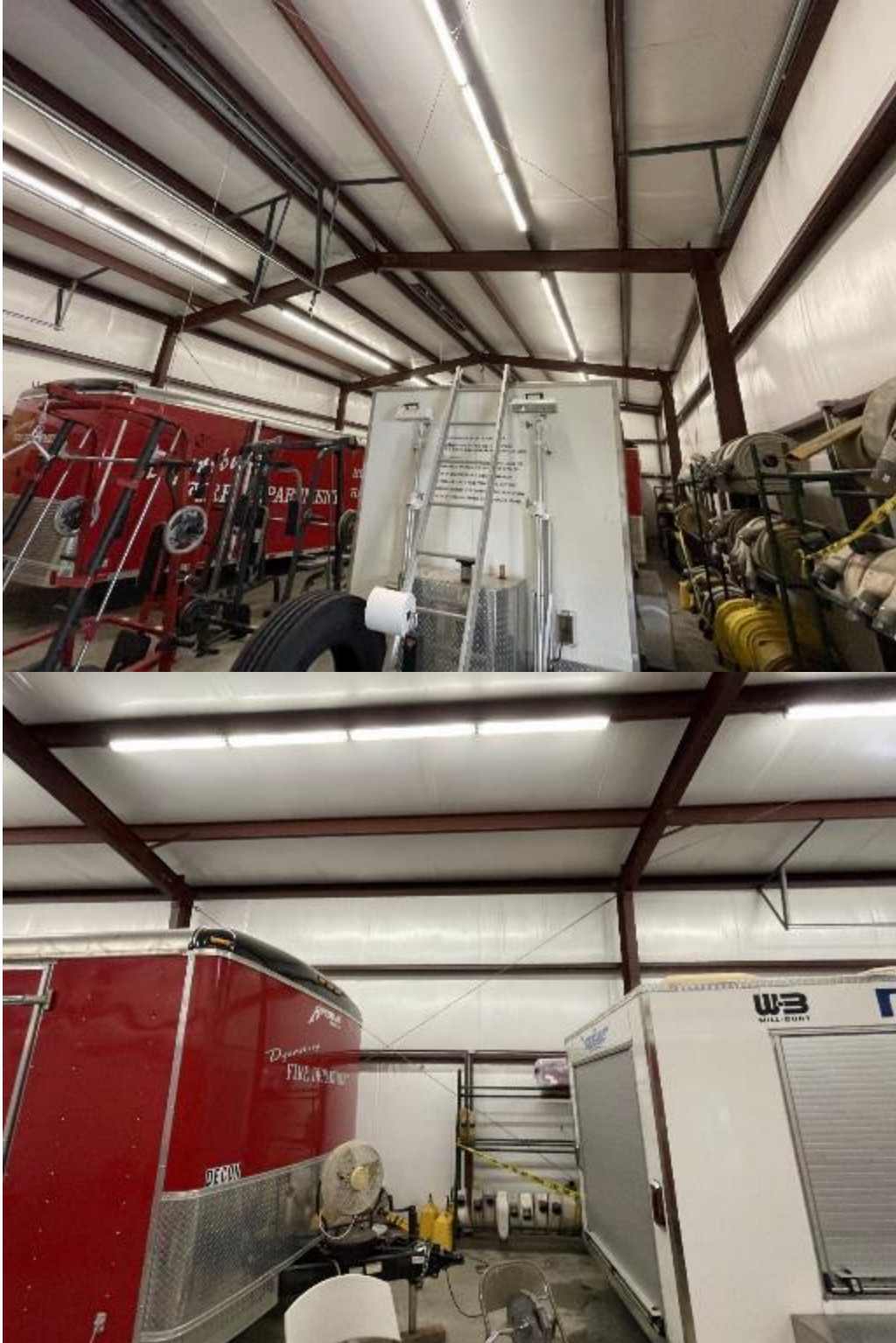
Figure J.23 Image of Structure #19.2
