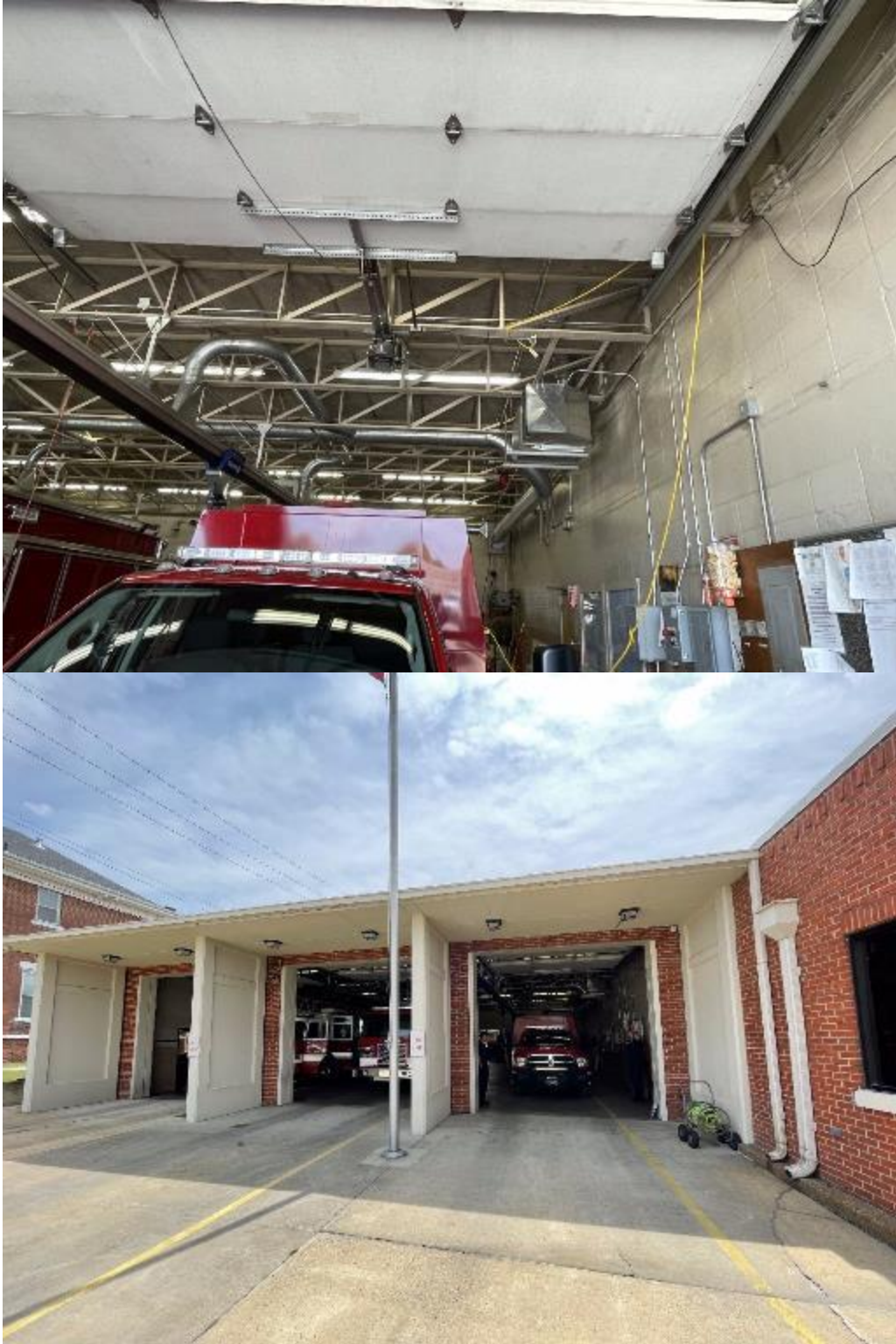
Figure J.31 Image of Structure #22
