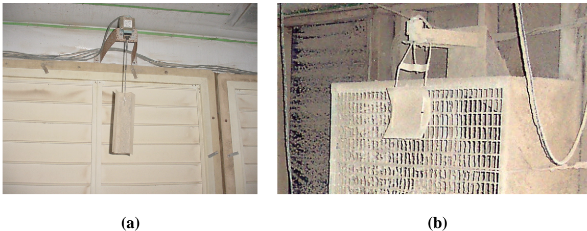
Figure 6. Initial sail switch arrangement used in North Carolina.
