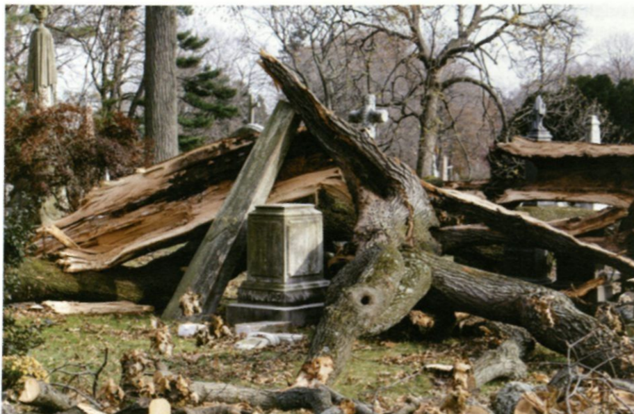
Figure 5.3. Hurricane Sandy damage in Green-Wood Cemetery Frederick Piccarello
