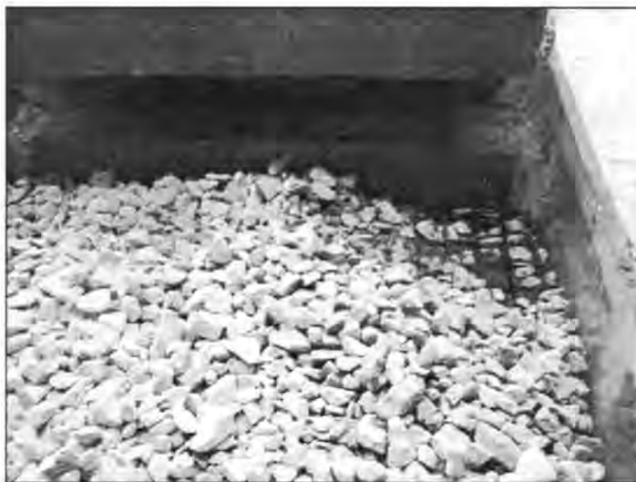
Figure 3.286 - Geogrid Placed under Special Backfill
