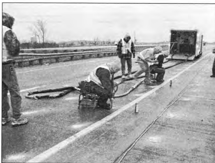
Figure 3.181 - Injecting High Density Polyurethane under the Approach Slab (Bridge No. 76.8065)
