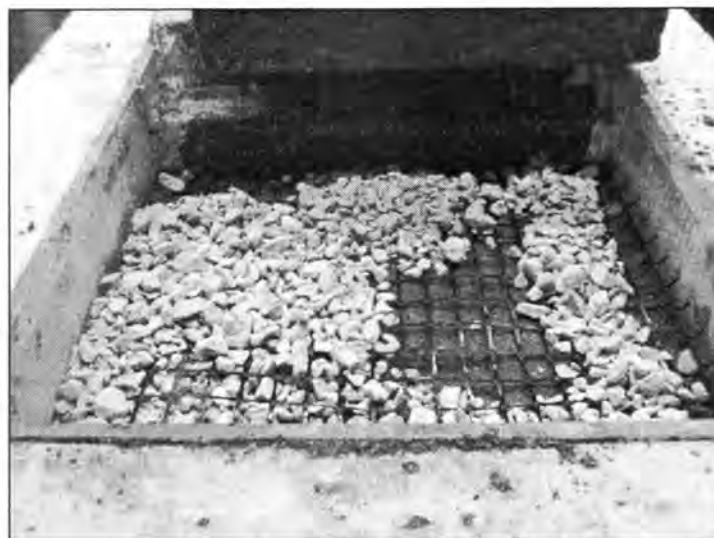
Figure 3.289 - Placing Special Backfill over Geogrid
