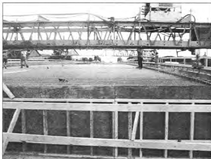
Figure 3.153 - Construction of Bridge Deck (Euclid Avenue Bridge)
