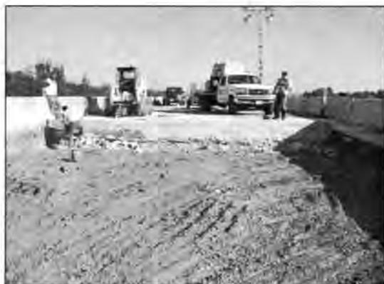
(a) Replaced Approach Slab
