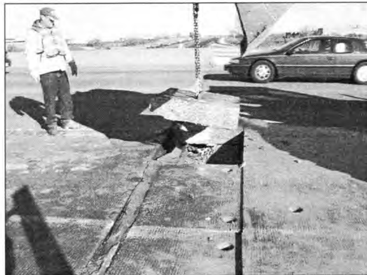
Figure 3.31 - Removing a Segment of the Approach Slab (Bridge Carrying 160 over I-35)
