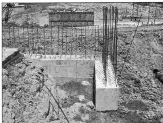
(a) Backwall construction
