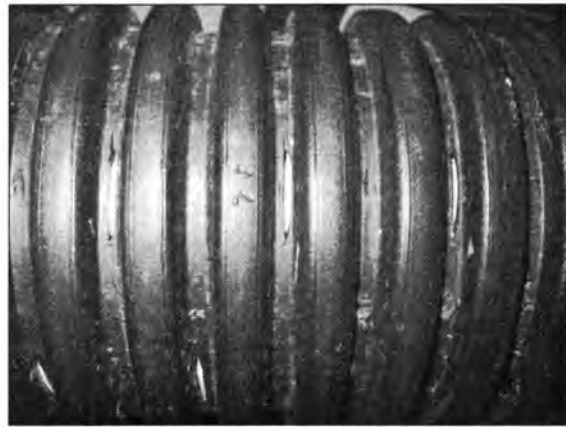
(b) Closer View of Pipe Openings
