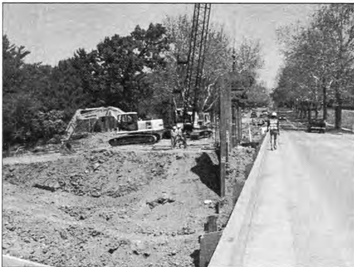
Figure 3.128 - Installation of the Sheet Piles (Polk Blvd. Bridge - NBL)
