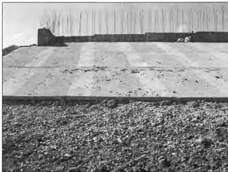
Figure 3.162 - Construction of Embankment Slope Protection (Euclid Avenue Bridge)
