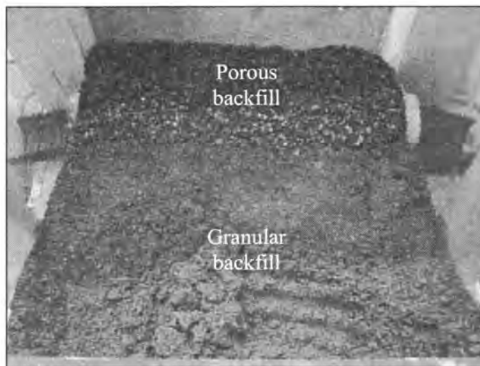
Figure 3.295 - Porous Fill Placed Around the Subdrain
