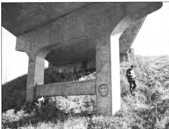
Figure 3.36 - Concrete Bridge with Deep Slab and No Girders (Bridge No. 1270.2S014)
