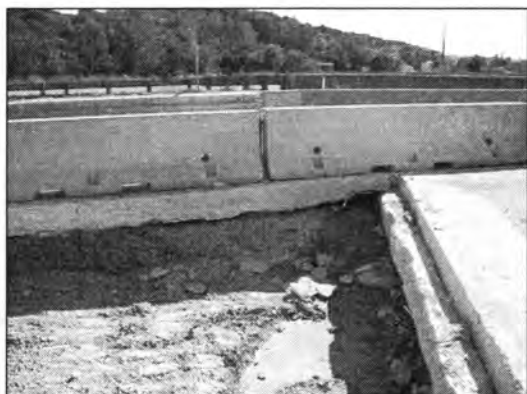
(a) North End Approach Slab
