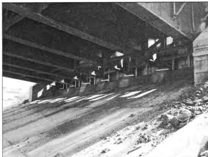
Figure 3.146 - Embankment Concrete Slope Protection (Pennsylvania Avenue Bridge)
