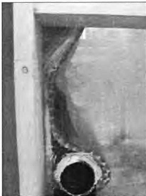
Figure 3.311 - Attaching the Geocomposite Drain to the Abutment
