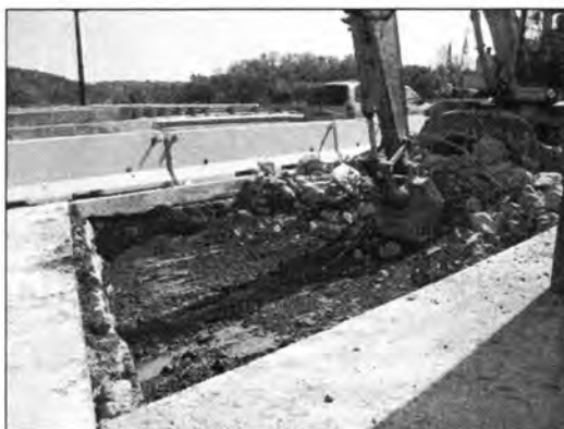
(b) South End Approach Slab
