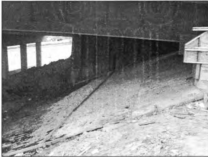
Figure 3.154 - Construction of Slope Protection at the Embankment (Euclid Avenue Bridge)
