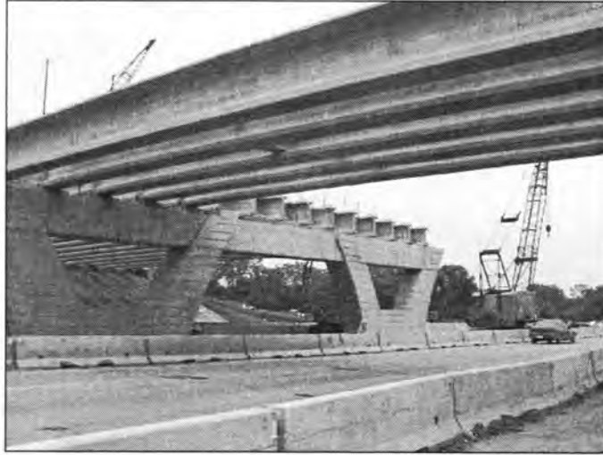
Figure 3.118 - Girders under Construction (35 th Street over I-235 - NBL)
