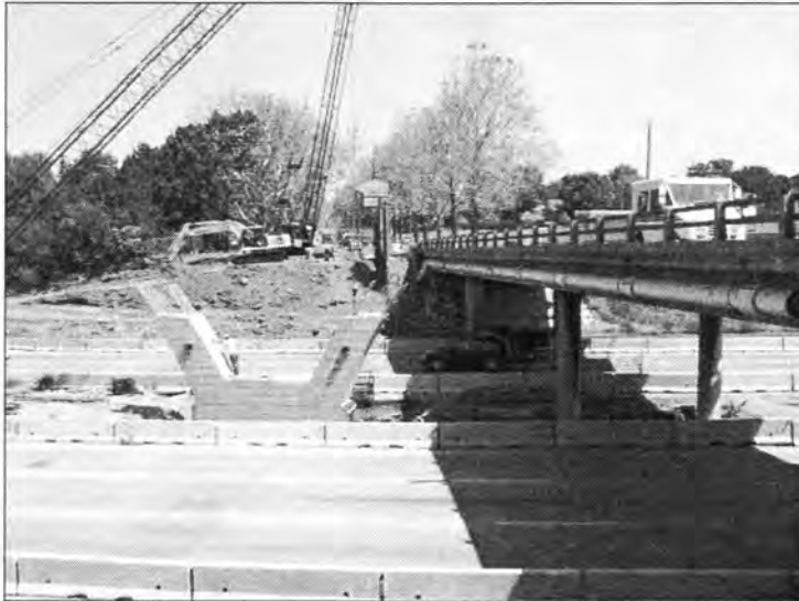
Figure 3.127 - Construction of the New North Bound Lane Bridge (Polk Blvd. Bridge)
