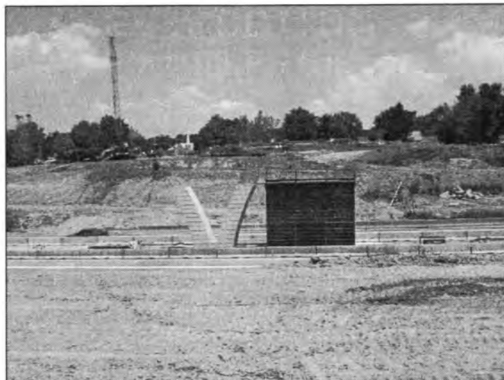
Figure 3.145 - Construction of Center Pier (Pennsylvania Avenue Bridge)
