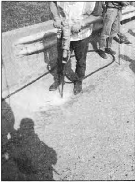
(a) Drilling at the Approach Slab
