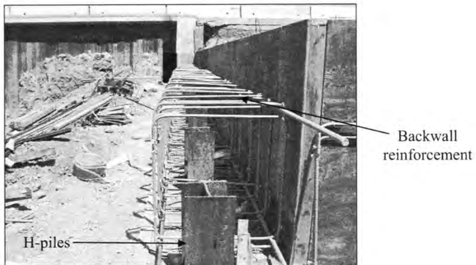
Figure 3.157 - Reinforcement for the Bridge Backwall (Euclid Avenue Bridge)
