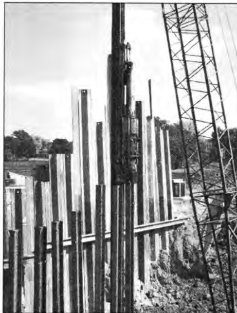
Figure 3.134 - H-Piles Being Driven Into the Ground (Polk Blvd. Bridge)
