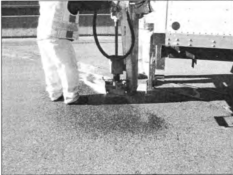
Figure 3.253 - Coring at the Bridge Approach (Bridge No. 7781.2065 - NBL)
