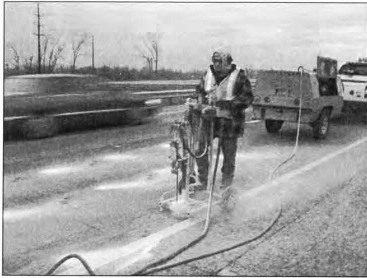
Figure 3.178 - Holes Drilled at the Approach Slab (Bridge No. 76.8065)
