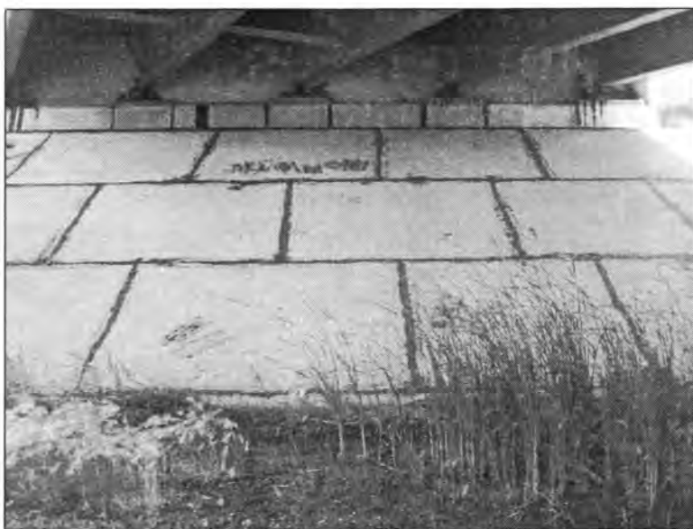
Figure 3.261 - Bridge Embankment in a Satisfactory Condition (Bridge No. 7782.8L065)
