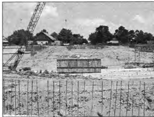
(b) Center pier construction
