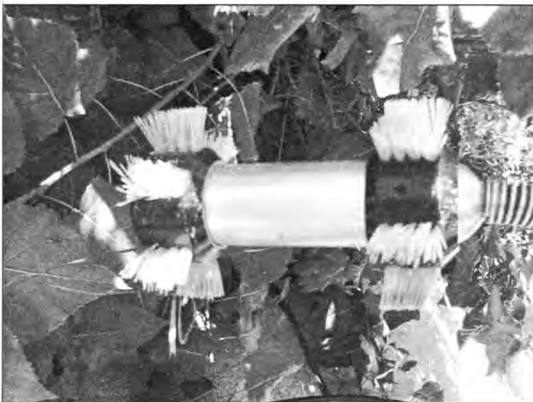
Figure 3.196 - Snake Camera used to Inspect Subdrains (Bridge No. 7773.0R065)
