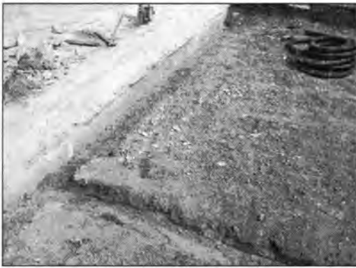
(a) Trench Excavated to Install Subdrain
