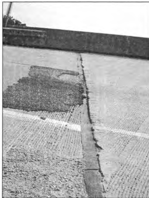
Figure 3.104 - Flexible Foam used as Joint Filler (Bridge No. 574.2S001)
