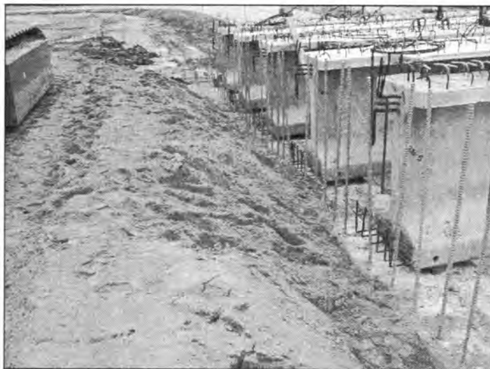
Figure 3.119 - Granular Backfill used behind the Abutment (35 th Street over I-235)
