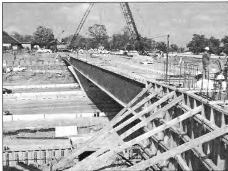
Figure 3.149 - Construction of Bridge Deck (East 12 th Street Bridge - NBL)
