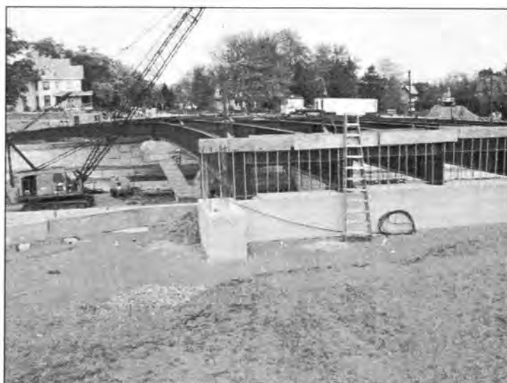
Figure 3.142 - Construction of Steel Girders and Backwall (19th Street Bridge)
