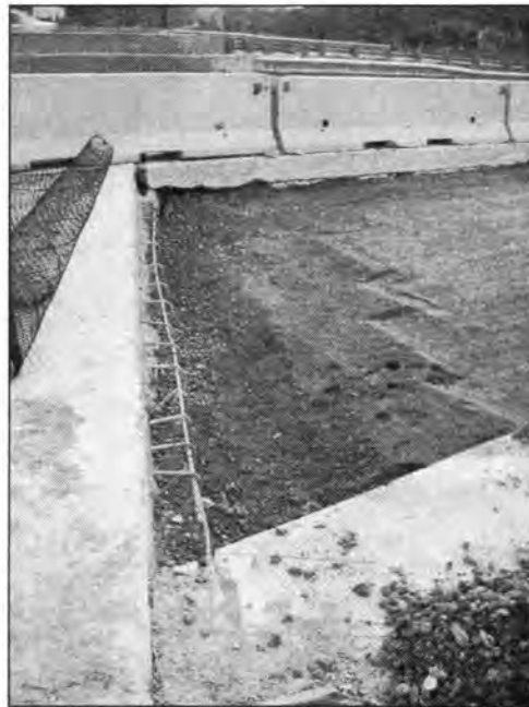
Figure 3.217 - Compacted sSocial Backfill (Bridge No. 7777.0R065 - South End of SBL)
