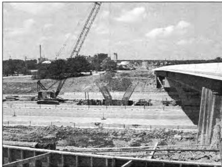
Figure 3.155 - Construction of the South Bound Lane Bridge (Euclid Avenue Bridge)
