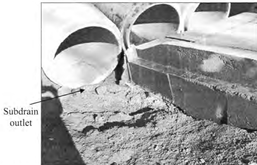
Figure 3.147 - Subdrain Outlet at the Bottom of the Embankment (Pennsylvania Avenue Bridge)
