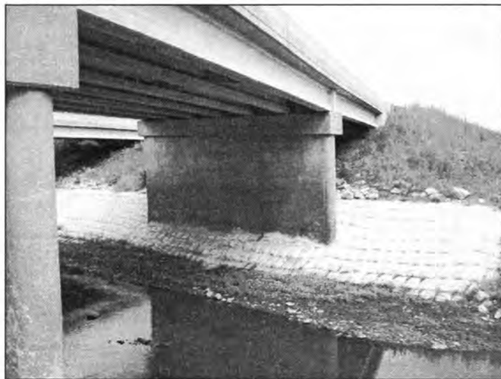
Figure 3.111 - Rocks and Pillows used for Embankment Stabilization (Bridge No. 5200.5R380)
