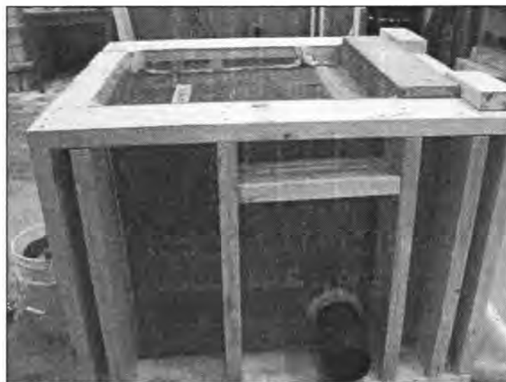
Figure 3.292 - Granular Backfill Placed behind the Abutment
