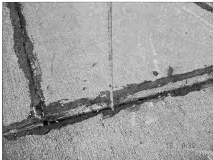
Figure 3.113 - Uneven Settlement of Slope Protection Panels (Bridge No. 5200.0R380)
