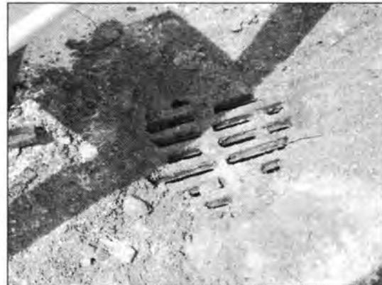
(b) Bridge End Drain After Debris Removal
