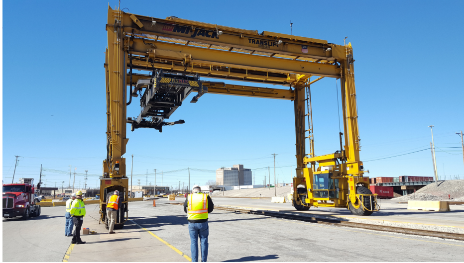
Figure 6.1: Gantry crane and crane way pavement.
