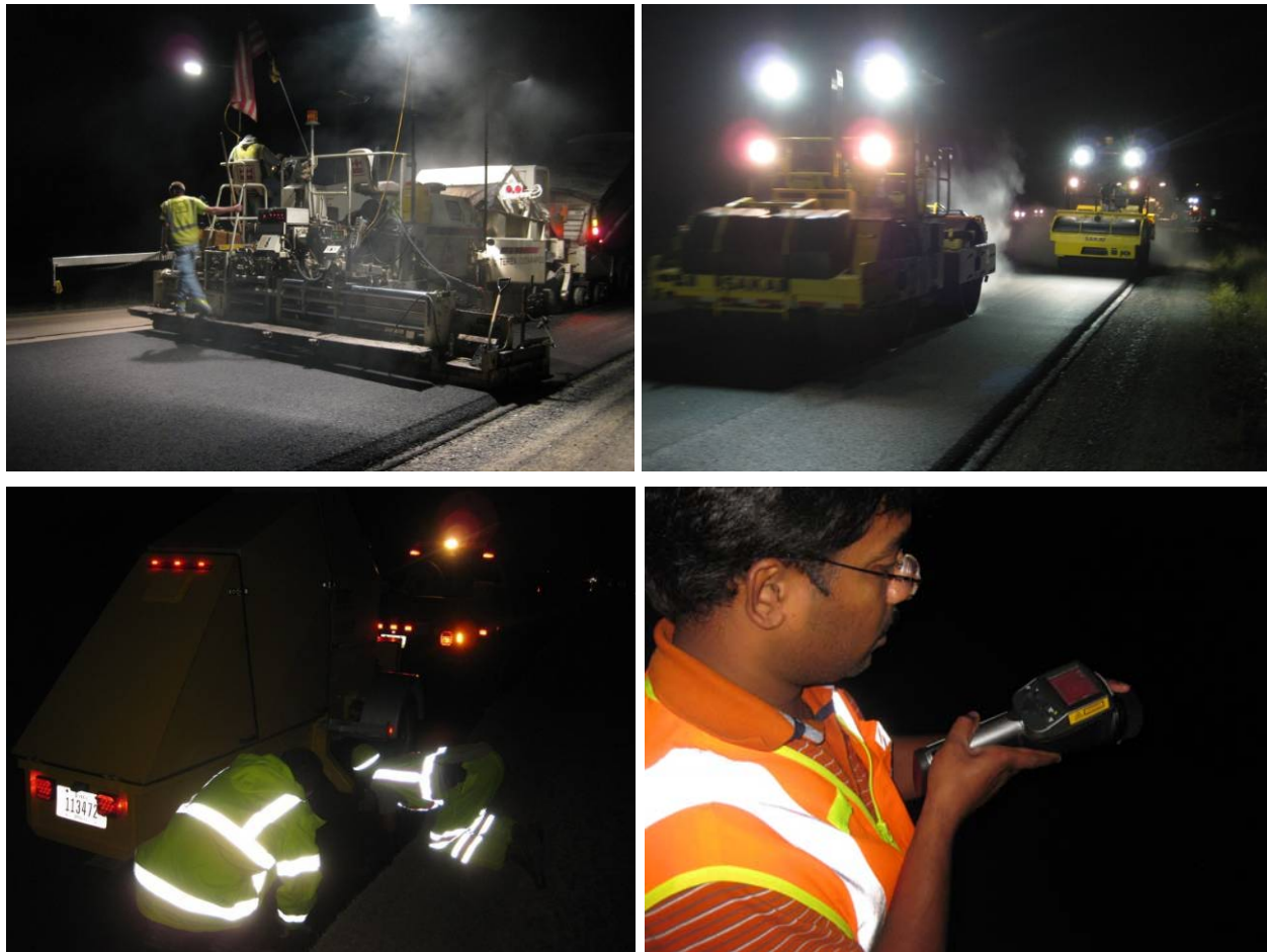
Figure 54. Photographs of paving operations and compaction, and in-situ testing
