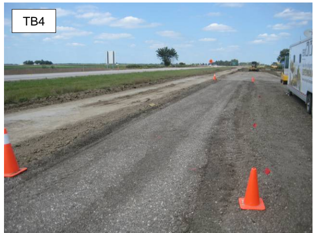
Figure 72. Photographs of special backfill subbase layer test beds construction
