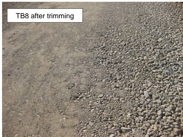
Figure 73. Photographs of aggregate base layer test beds construction
