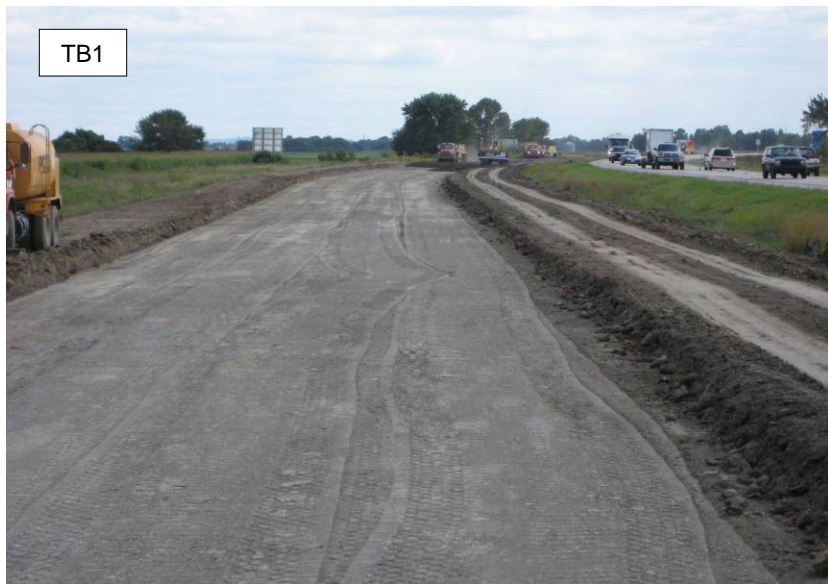
Figure 71. Photographs of subgrade test beds construction
