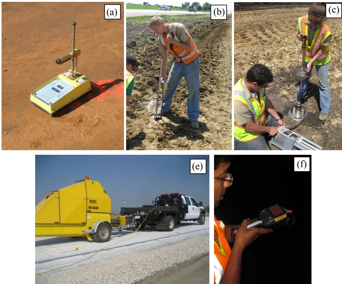
Figure 4. In-situ testing methods used on the project: (a) Humboldt nuclear gauge, (b) dynamic cone penetrometer, (c) Zorn light weight deflectometer, (d) KUAB falling weight deflectometer, (e) FLIR thermal imaging camera
