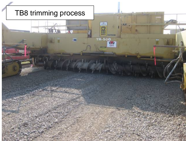
Figure 73. Photographs of aggregate base layer test beds construction
