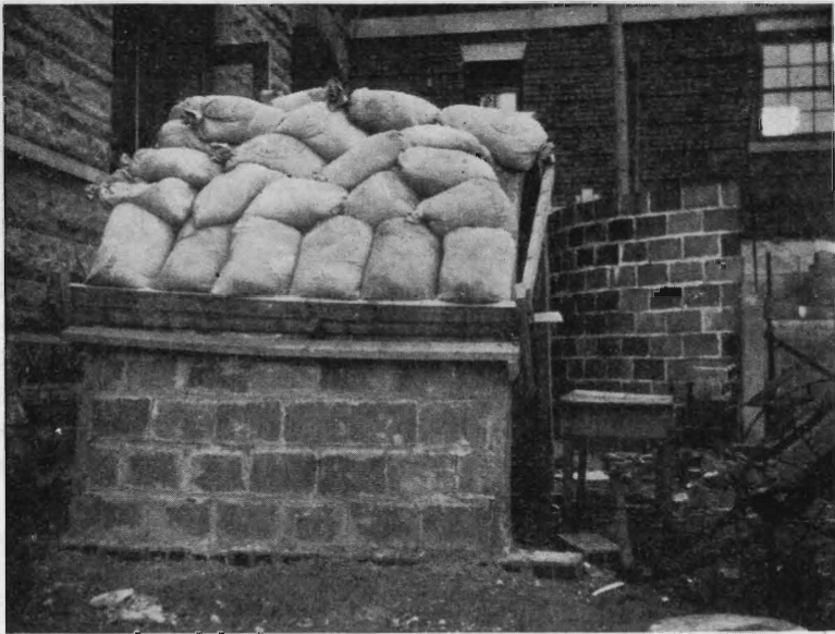
Fig. 8. Manner of loading the model roof for the strength tests.
