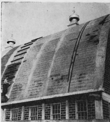
Fig. 34. Treating of the leaky areas with fibered asphalt and aluminum paint.
