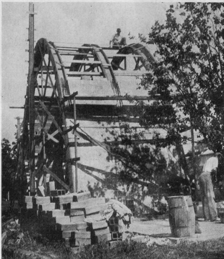
Fig. 25. Construction of the full sized arch roof section.
