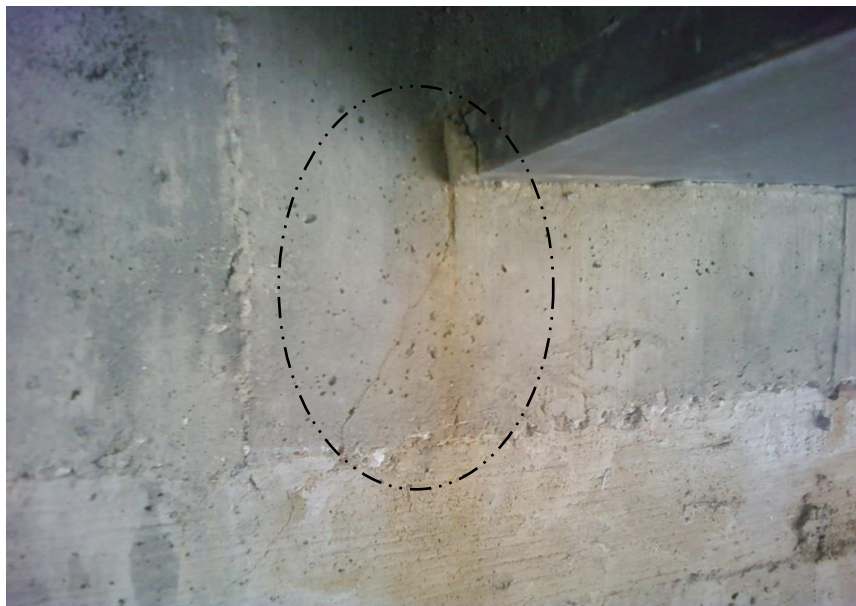
Figure 4.7. North abutment and bottom flange interface
