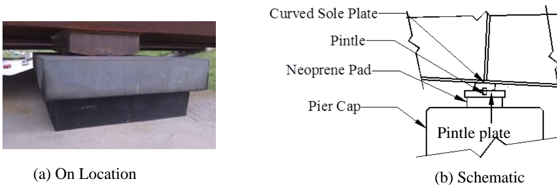
Figure 5.10. Expansion pier bearing
