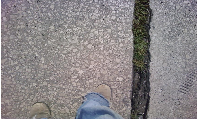
Figure 4.6. Approach slab/bridge joint
