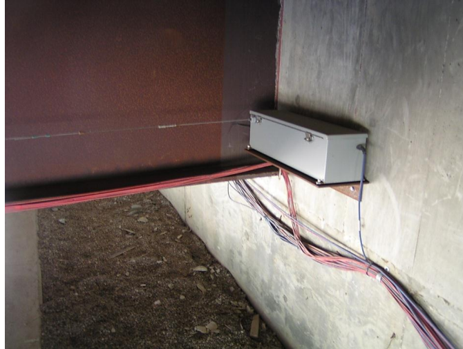
Figure 5.19. Long-range displacement meter
