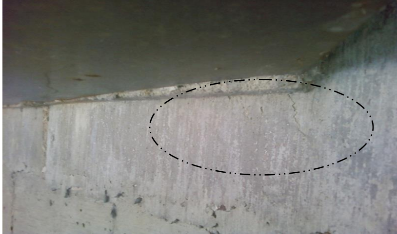
Figure 4.2. North abutment and bottom flange interface
