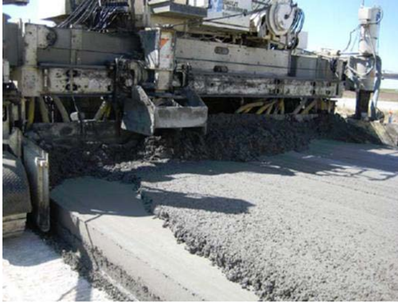
Figure 2-6 Two-lift construction of concrete pavement in progress (Hu et al. 2014)
