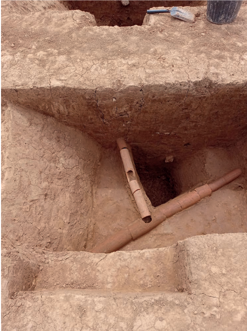
Fig. 12. Photo showing drainage pipes in slot 4
