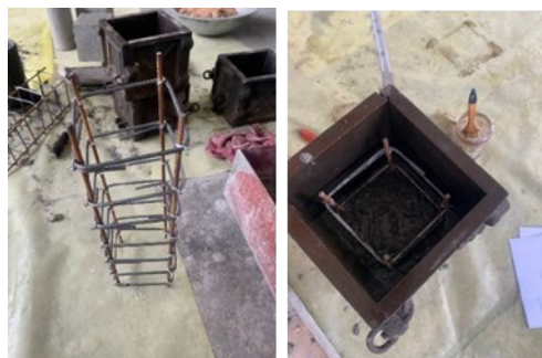
Fig. 3: Steel reinforcement of RC columns.
