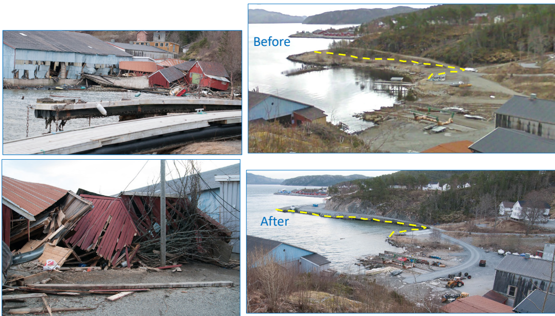
Figure 3.1 Photos showing damage caused by the Statland landslide. The right hand side photos compare the situation before and after the landslide.
