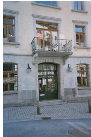
Figure 21. Town hall of Salvan (Source NF1)
