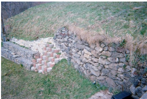
Figure 11. Different techniques for levelling the soil (Source NF7)
