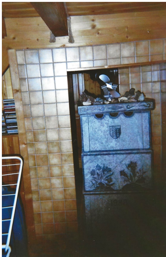
Figure 33. Furnace to heat up the house with wood (source P1).
