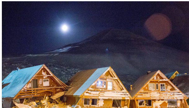
Figure 4. Damaged houses after the avalanche December 2015 [15] (photo: Geir Barstein)
