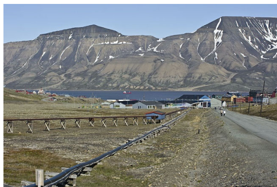
Figure 10. Piping over the ground on permafrost [24].
