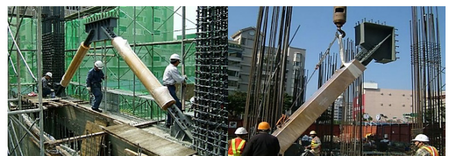
Fig. 2 BRB installation in RC frames
