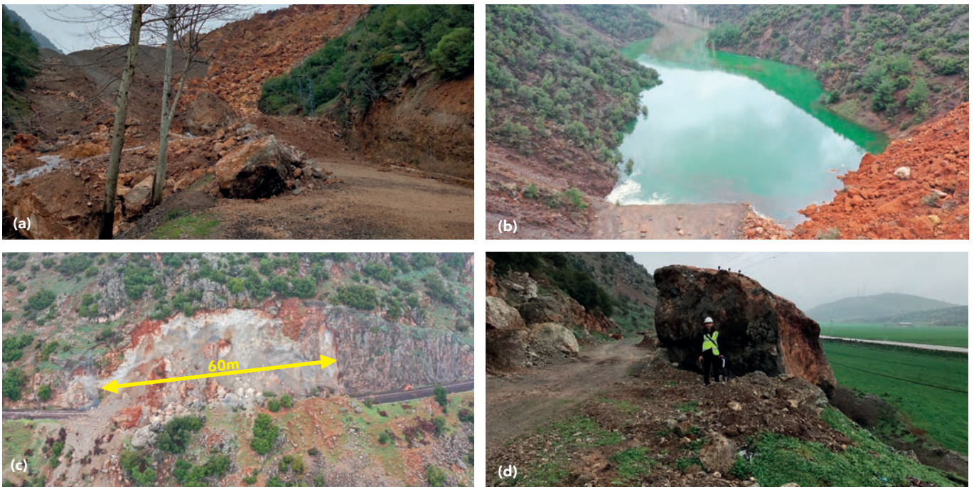
Figure 1: Landslides and rockfalls close to Islahiye
