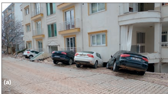
Figure 4 (above): Liquefaction and subsidence in İskenderun
