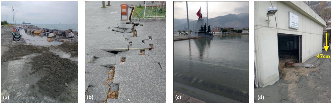
Figure 3 (above): Liquefaction and subsidence in İskenderun
