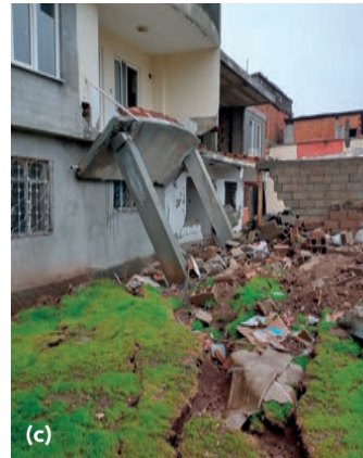
Figure 2: Surface feature interaction with buildings in Gölbaşı, Adıyaman. All photos were taken along the same rupture feature
