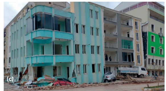
Figure 5 (left and right): Liquefaction-related failures in Gölbaşı
