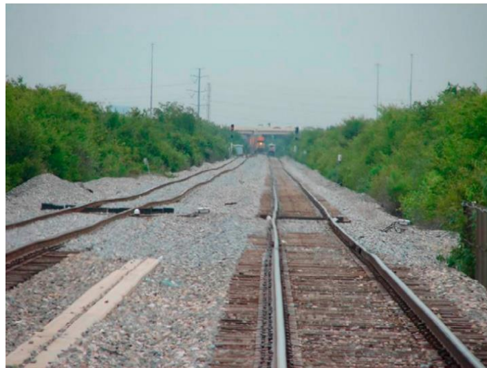
Figure 2.0-6. Example of track geometrical VLL in a ballasted railway track (Lazorenko 2019).
