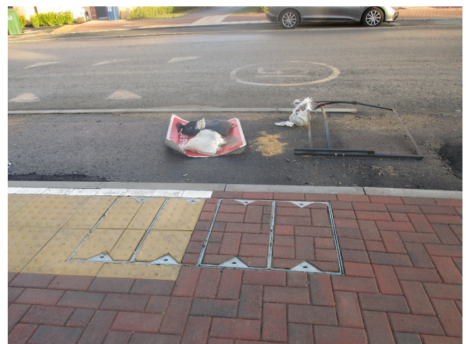
Fig. 2. Debris on the bike path
