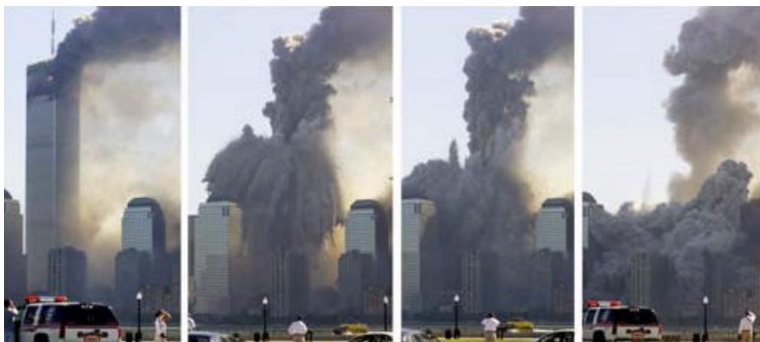
Figure 2. 9 World Trade Centre pancake type progressive collapse (Clifton, 2001).
