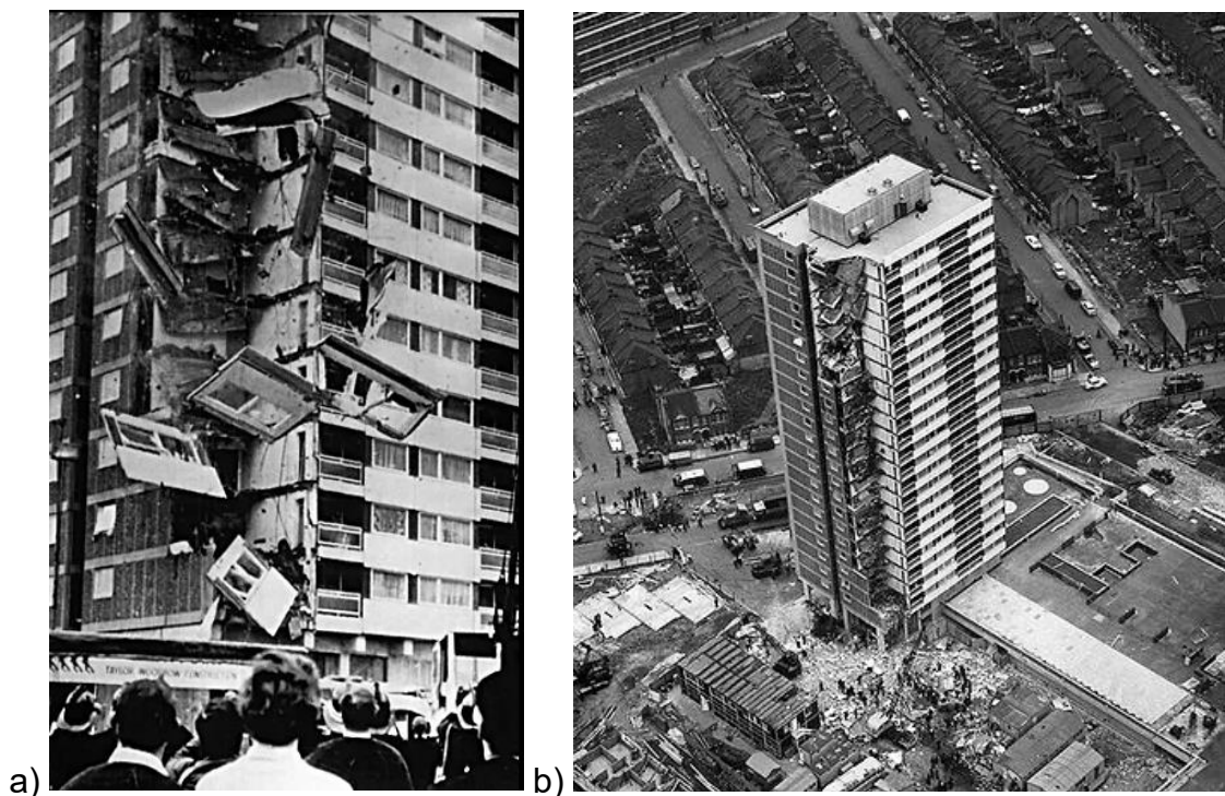
Figure 2. 7 Ronan Point collapse (a) during and (b) after the collapse
