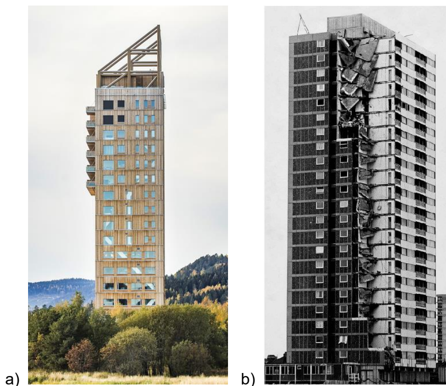
Figure 1. 1 (a) The Mjøstårnet Tower (photo by Ricardo Photo ©) and (b) Ronan Point progressive collapse extracted from Palmisano, (2014)
