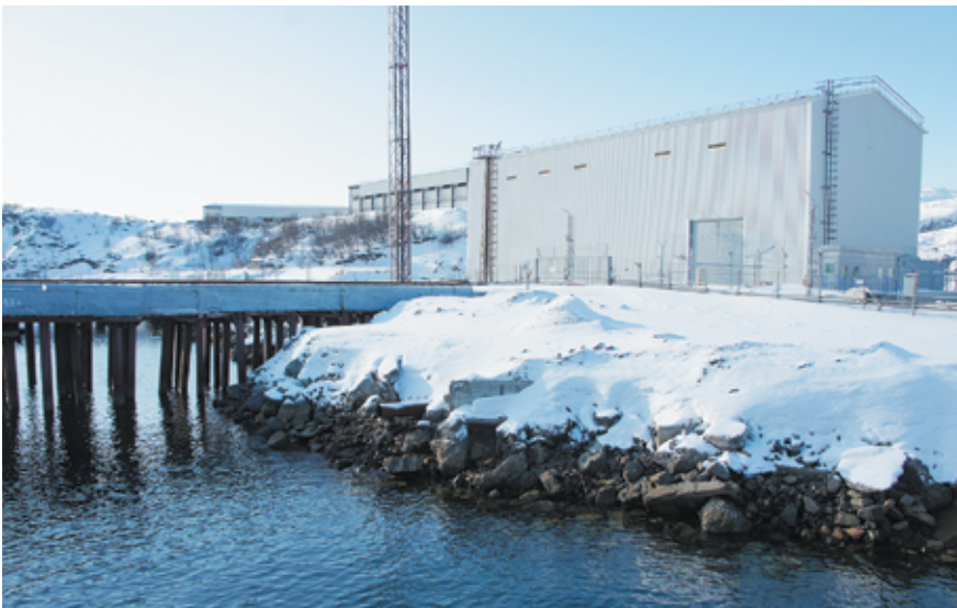
Infrastructure units built in Andreeva Bay with the help of international donors, 2014. Photo from the Bellona archive.
