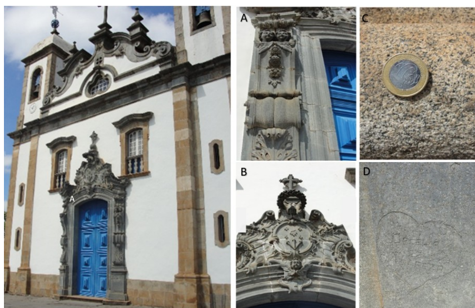
Figure 3: Features of the Bom Jesus de Matosinhos Church's facade. The granite is present in the base columns and bell towers, while the soapstone occurs in the doorway (A), cornice, oculus, cross and ornaments (B). Note the yellowish color of the granite due to the presence of patina and dust (C) and the depredation with an inscription on the column (D).
