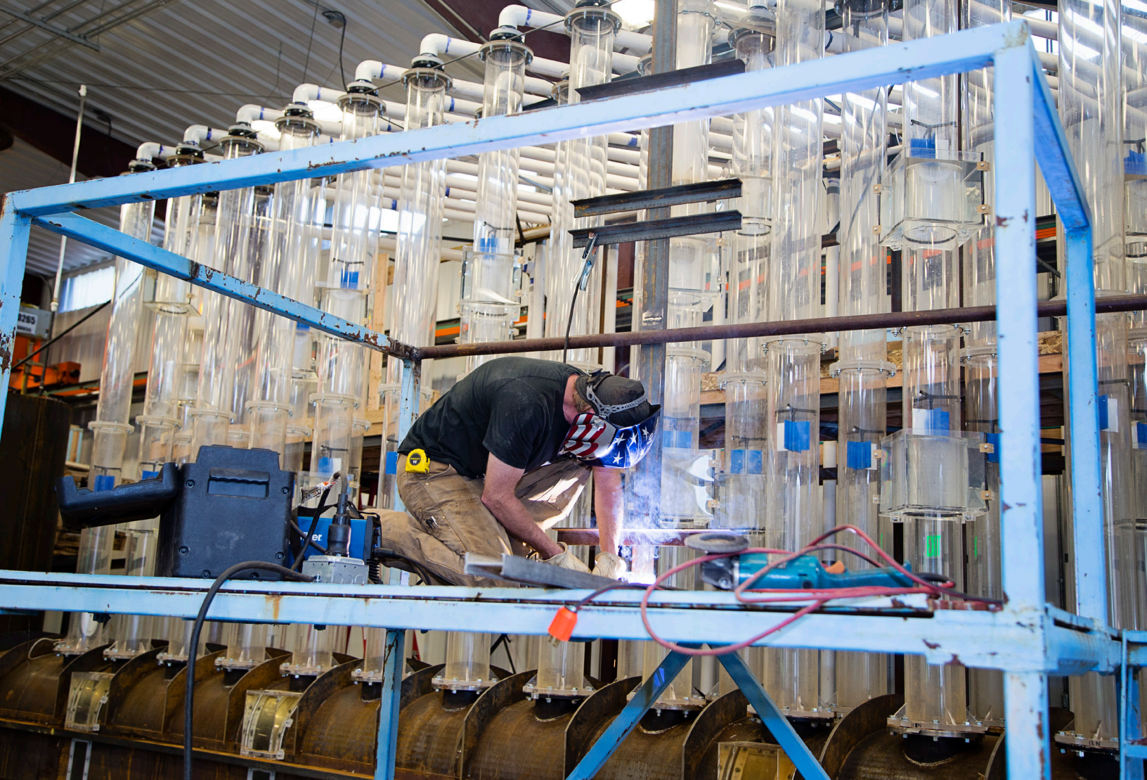
Research Engineer Andy Lee helped build the pump station scale model inside the UWRL's Hydraulics Modeling Lab.
