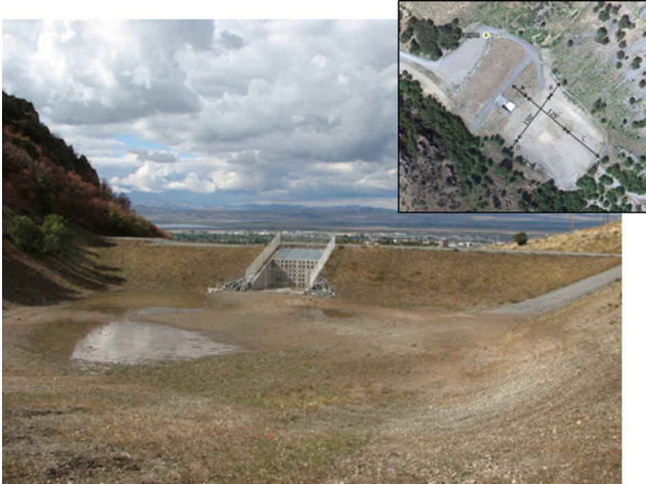
Figure 23. Looking west out of the mouth of the Dry Canyon detention basin (main). Aerial view of the Dry Canyon detention basin (insert).
