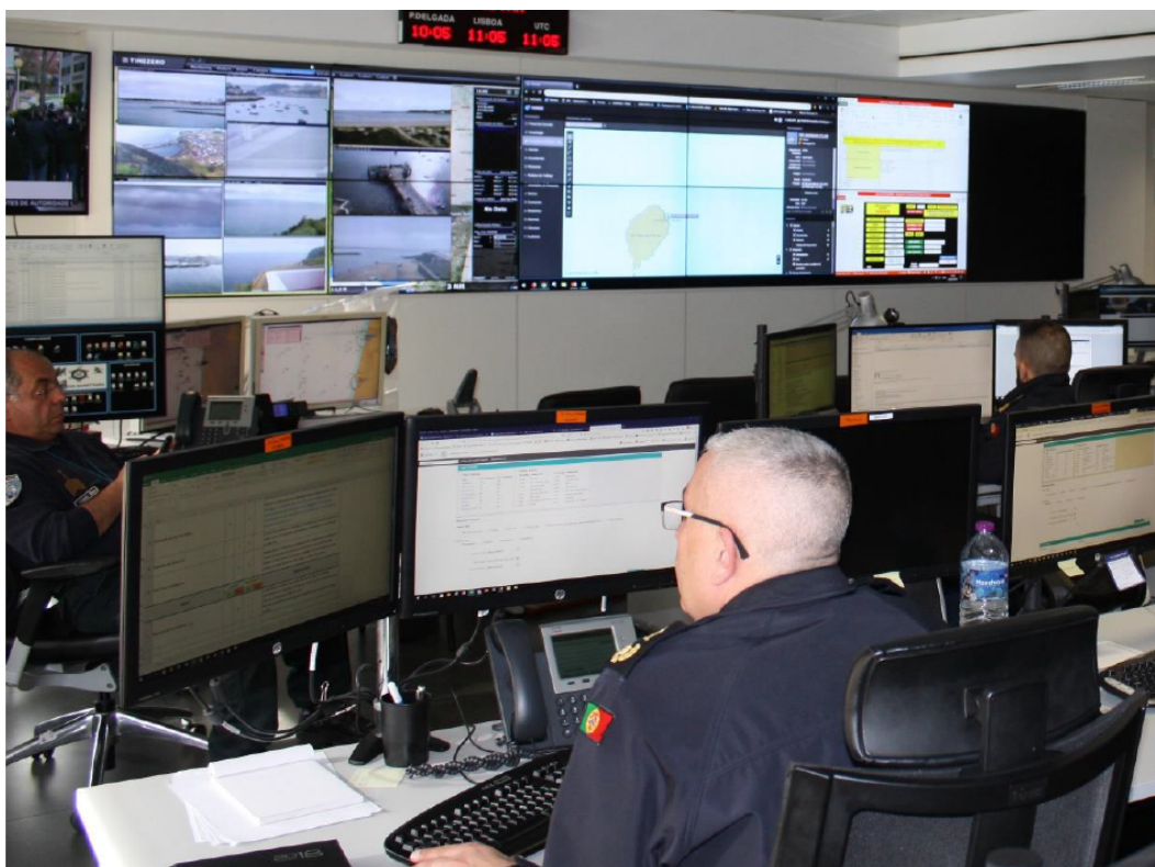
Figure 2.4: Maritime Operations Centre in Portugal using a release version of OVERSEE
