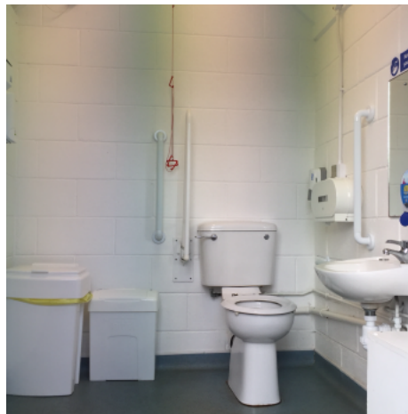
Figure 1.2: Pull cord placed next to a toilet. If the elderly falls outside the bathroom, this alarm would never be activated [10].
