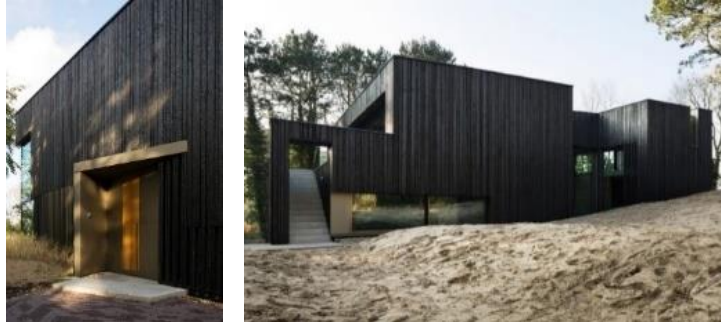
Figure 6. Villa Meijndel in Netherlands used Shou Sugi Ban finishing on the outdoor wall building [Source : Griffiths [9]]
