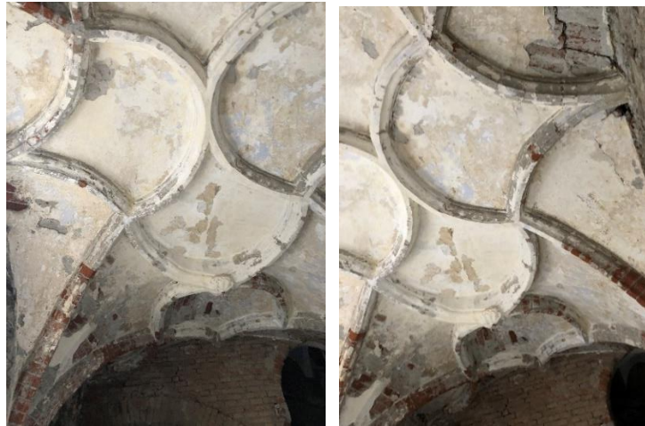
Fig.3 – Inside the house No.12, Jáchymov, year 2021. Gothic ribbed circular vault.
