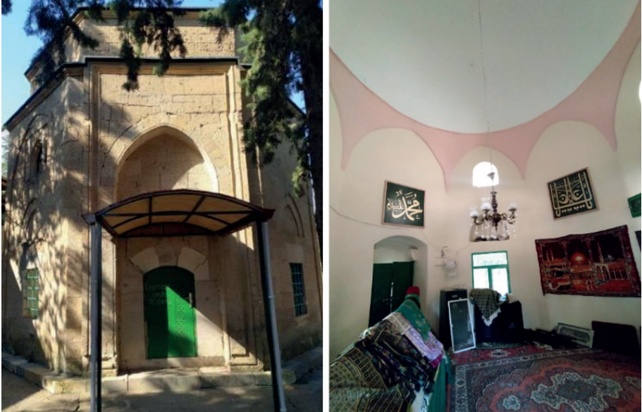
Figure 16. The Entrance Facade and Interior of the Tomb
