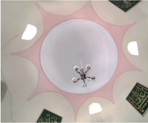
Figure 17. Ceiling covering in interior
