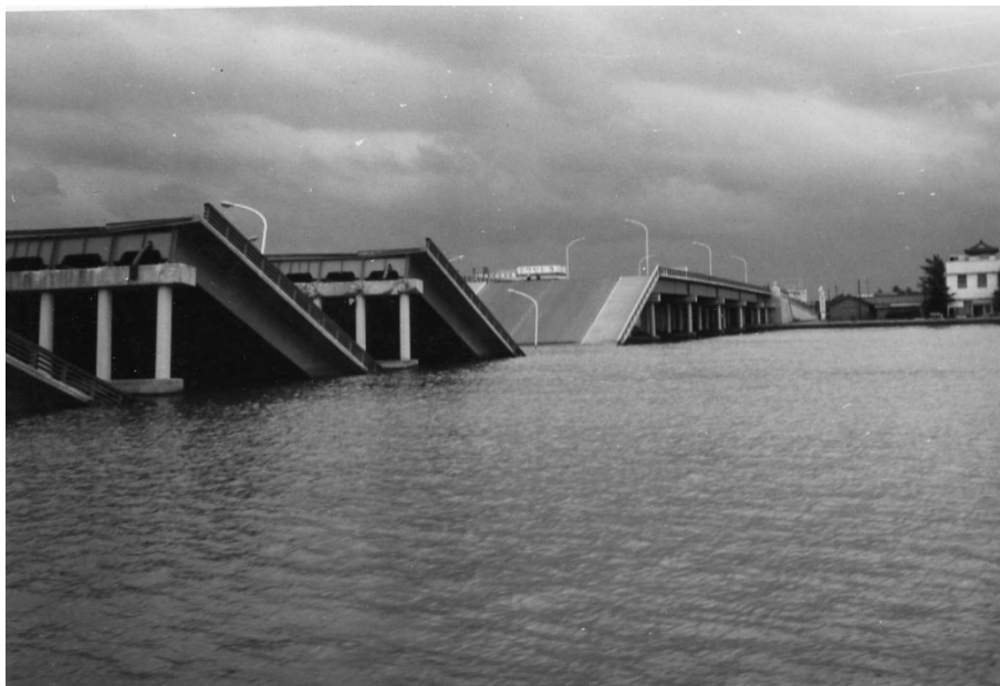
Fig. 1.1. Collapse of Showa Bridge due to liquefaction after the 1964 Niigata earthquake (Photo: Photographs and motion picture of the Niigata city immediately after the earthquake in 1964).
